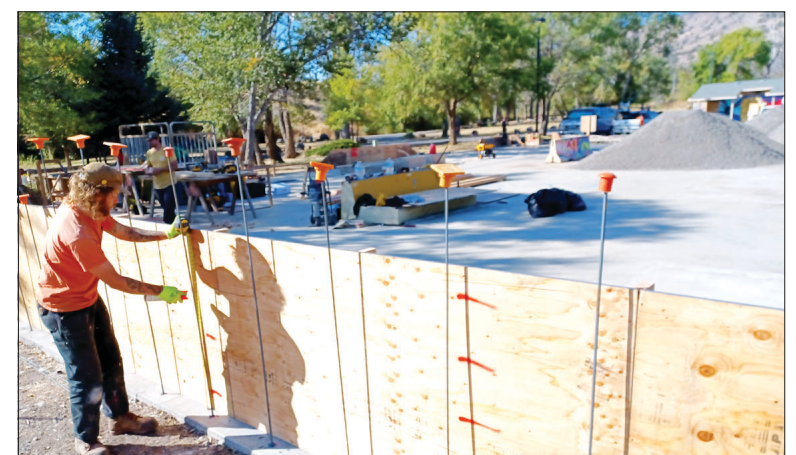
Skatepark construction this week at Elmer Quinn Park.
