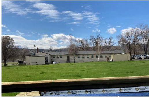
The old school cafeteria served students at Warm Springs Elementary for many years. The facility is currently being remodeled for multiple purpose use including a commercial kitchen.
