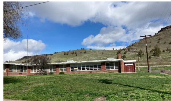
The old Warm Springs Elementary School was added on to after the older section of the school outgrew the need to accommodate more students. Currently this building is not in use beyond storage for Emergency Operations while assessment are being done for abatement, remediation and renovation. Students moved to the new K-8 Academy in 2014.
